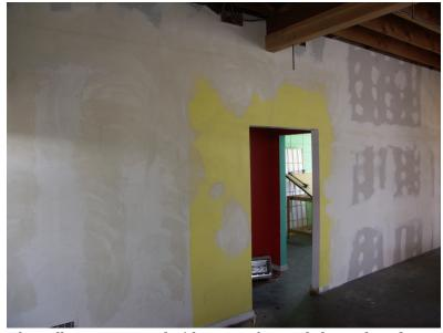
The walls were prepared with a coat of natural glue and sand
