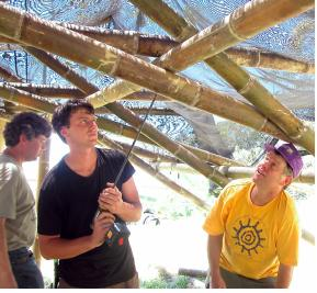
Drilling holes through multiple bamboo poles requires a steady hand and extra eyes. Ideally the bolt passes through at the exact intersection of adjacent poles. This will allow for the most even distribution of loads while offering the cleanest aesthetic. After drilling the holes it is wise to place the threaded rod immediately to avoid misalignment later.
