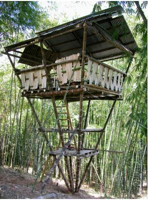
Jo Scheer designed and led the building of this mid canopy observatory as part of the outdoor lab project. The Structure also known as a Hooch is tied off to surrounding bamboo plants. Its design is stable, but allowed to move in the breeze.
