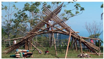
With the skeleton in place the crew moved on to creating the final connections using threaded rod and cement mortar.
