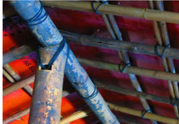
A typical pillar to ridge beam connection, demonstrating consistent and quality craftsmanship.
