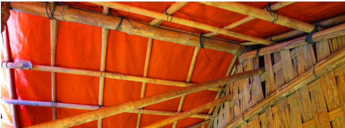
Method B: The bamboo rafters provide the primary support of the roof tarpaulin. This reduces potential for rainwater pooling because any draping of the tarp slopes continuously to the eave. The purlins are whole round Mulli bamboo, and
