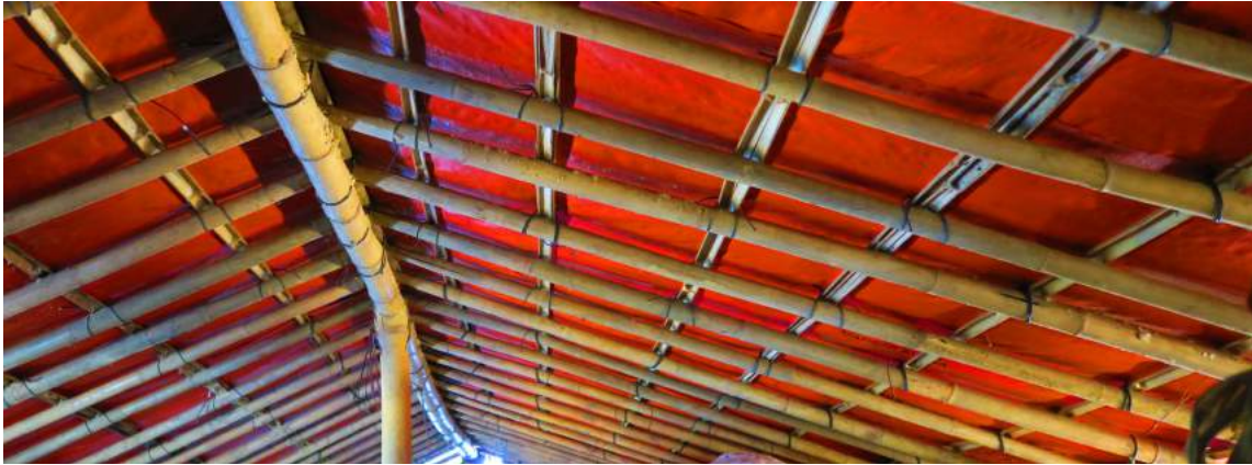
Method A: The purlins provide the primary support of the roof tarpaulin. In this variation the purlins are split Mulli bamboo with the cun side down, lashed to and supported by the bamboo rafters.
