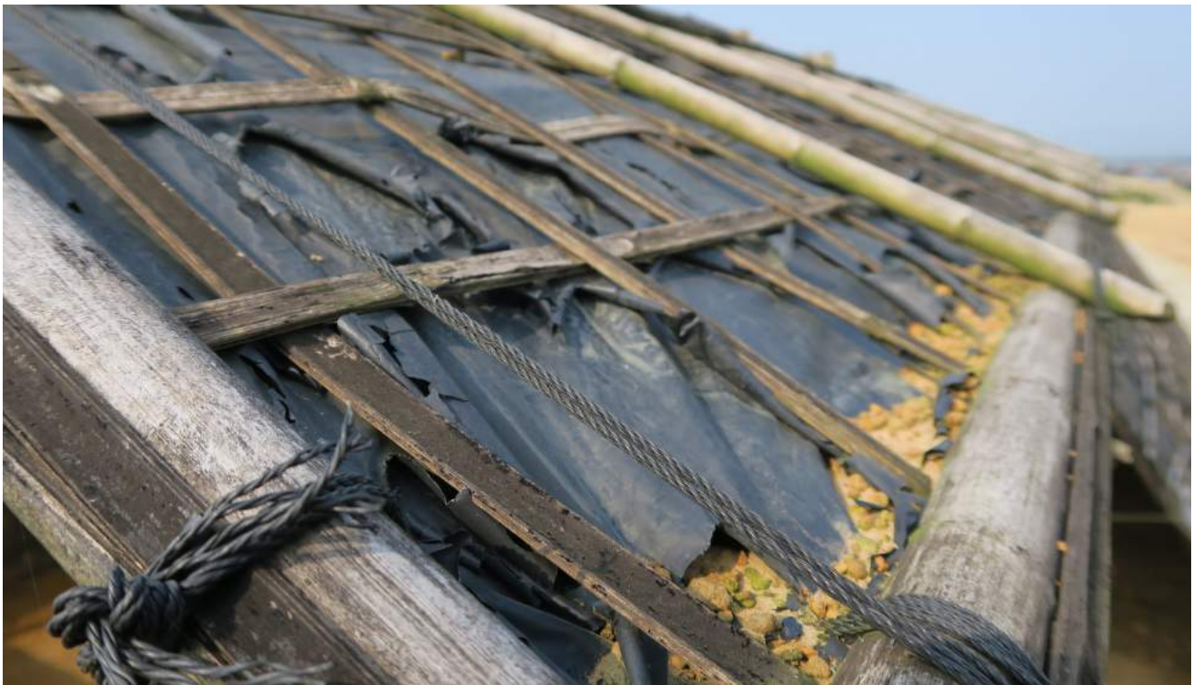
A close up of a roof shows the deterioration to the top layer of black plastic, the small amount of earth on the bottom edge is washed down from a sandbag put on the roof during the rains. The sandbags helped to reduce the uplift on the membrane during winds. This is an owner implemented innovation.
