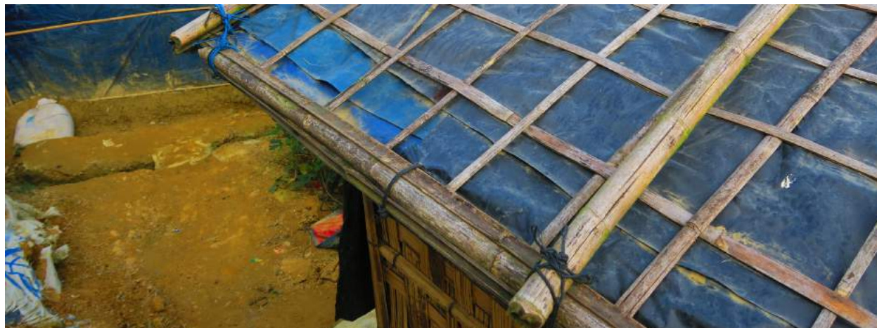
This exterior view of the roof edge shows typical exterior battens, rafters and roof edge lashings, all of which protect the tarp from wind damage.
