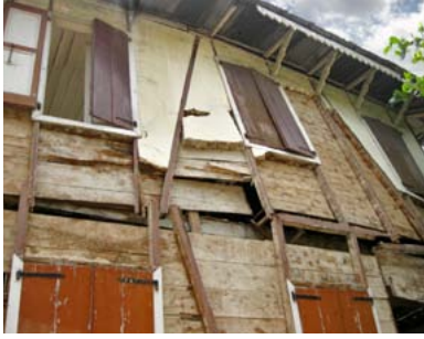
FIGURE 123 Typical vulnerability: the wall pulls away on the side parallel to the floor framing due to lack of connectivity between the floor and the wall. This is easily improved in most houses.
