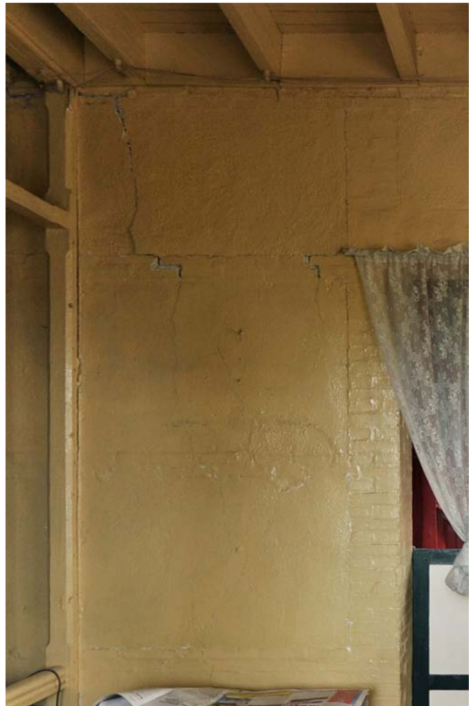
FIGURE 128 Interior and exterior examples of low levels of damage to rubble stone panels in masonry walls.
