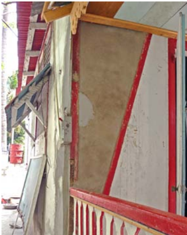
FIGURE 135 Well-intentioned but improper repairs with cement mortar in brick work ( above and right ), and cement plaster for colombage infill ( below ). Lime mortar and lime plaster should be used.
