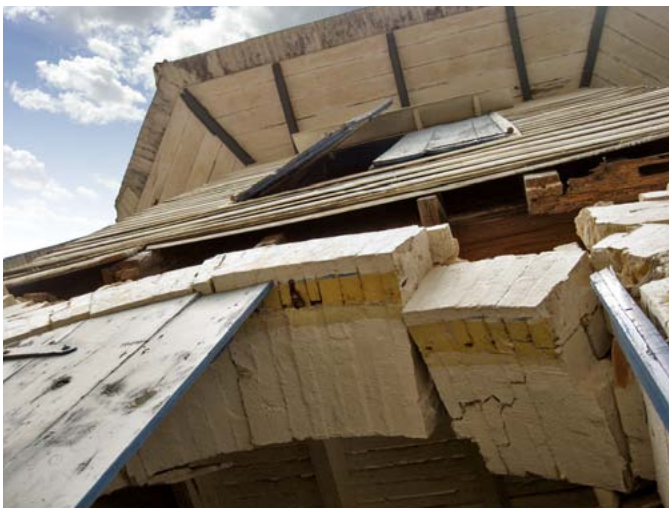
FIGURE 105 Severely damaged arch, and displaced wood framing above. Absence of tie rods, combined with decay of the timber sill plates made the building more vulnerable.
