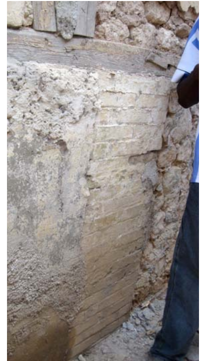
FIGURE 51 The original brick masonry foundation pier can be seen and is infilled on either side with stuccoed stonework. Rising damp from the ground has caused extensive deterioration to the exposed stone masonry. This results from the migration of soluble salts to the surface where they expand on drying, causing the surface of the masonry to spall.
