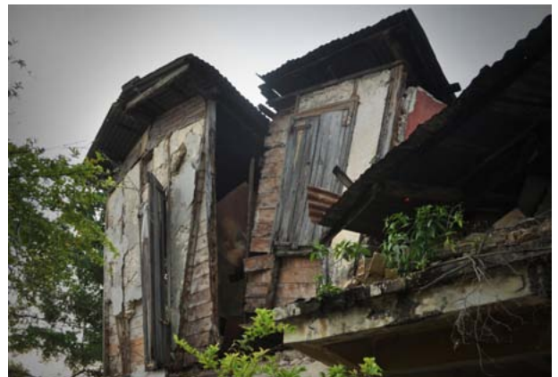
FIGURE 63 Heavily rotted and termite-eaten house on Avenue Lamartiniere, which partially collapsed during the earthquake.
