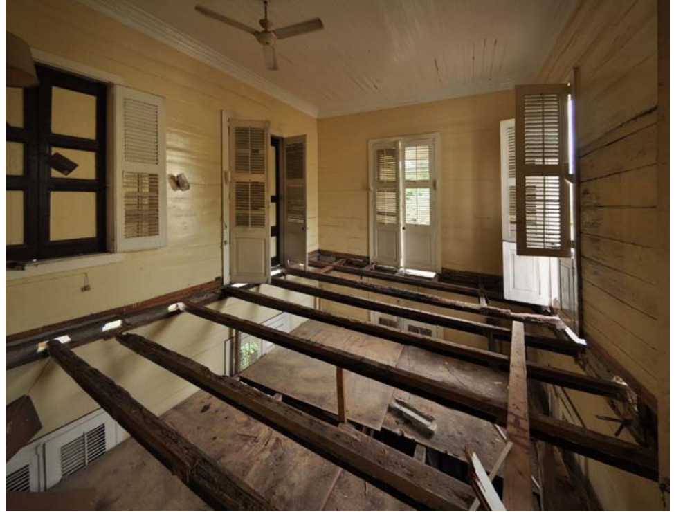
FIGURE 124 House at 32 Avenue Lamartiniere now under restoration, showing the decayed ends of the joists.
