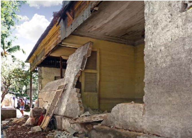
FIGURE 72 A replacement side wall of concrete block at 19 Lamar-tiniere suffered partial collapse.
