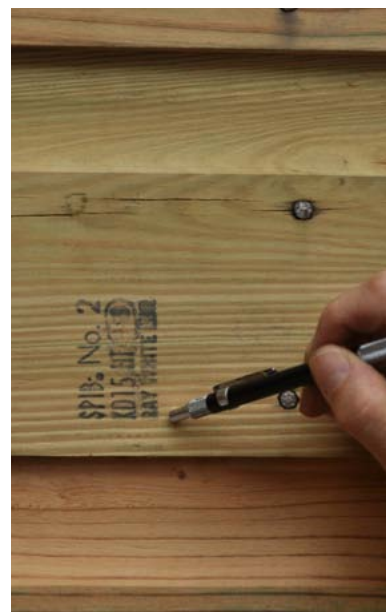
FIGURE 126 Owner and architect Gilbert Mangones explaining the restoration work he is doing on his house at 24 Avenue Lamartiniere, shown in Figures 24, 35, and 134. The new ship lap siding is pressure treated imported timber. The timber grade stamp is shown below.
