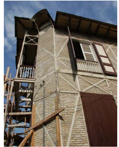
FIGURE 42 The house at 32 Lamartiniere. The braced timber frame and brick infill is a large component of the architectural vocabulary.
