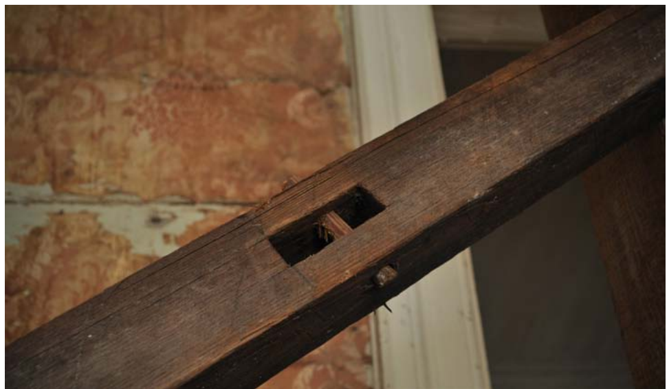
FIGURE 32 top The interior of a room constructed on what had been the porch of the Patrice Pamphile House at 4 Rue Casseus, shown in Figure 2. This interior shows the characteristics of the typical timber frame construction in Haiti, which lies somewhere between the heavy timber framing with mortise and tenon jointing common in Medieval and Renaissance French construction, and the sawn light timber “balloon frame” of nineteenth-century American construction. bottom This example of a mortise and peg is from the Bazin House at 8 Rue du Travail Deuxième.
