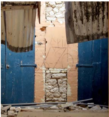
FIGURE 46 Characteristic ‘brick frame’ with rubble infill construction
