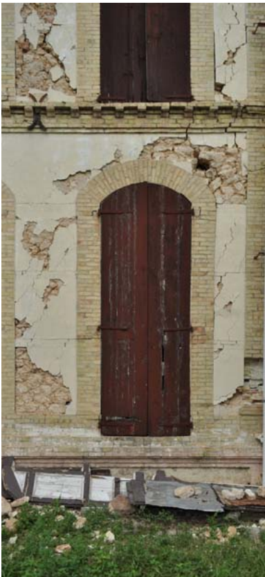
FIGURE 127 Typical 'brick frame' with rubble infill construction. Note crack pattern/energy absorption in rubble fill. The addition of ties to resist the spreading of the arches at the tops of the openings will improve earthquake resistance, especially when the arch is close to the corner of the building as in the figure on the left.
