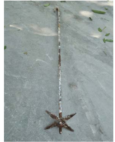
FIGURE 101 Iron chains are common in many of the masonry walls of the Port-au-Prince Gingerbread houses. Above is the first section of the chain with the star-shaped metal plate, and the view at left shows the metal plates where they remain holding the wall at the floor level in place, thus stopping the further separation of the walls at the corner. Had these floor level reinforcement rings not been installed, the lower floor walls would probably have collapsed as well.
