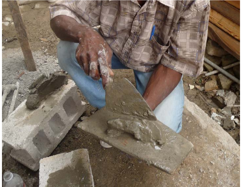
FIGURE 135 Well-intentioned but improper repairs with cement mortar in brick work ( above and right ), and cement plaster for colombage infill ( below ). Lime mortar and lime plaster should be used.
