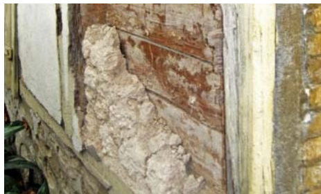
FIGURE 87 Close-up view of the failed colombage stonework. This infill, if laid up in clay, crumbles away and does not compromise the integrity of the wood braced frame.
