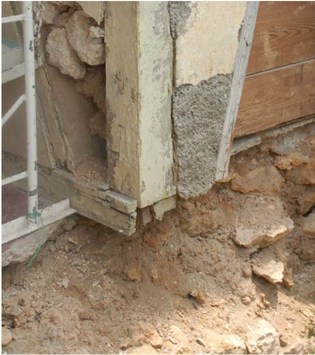
FIGURE 79 The wood sill that was previously termite damaged was crushed during the earthquake. This caused the entire structure to settle on its foundation. The result is that many of the doors to the exterior cannot be opened or closed.
