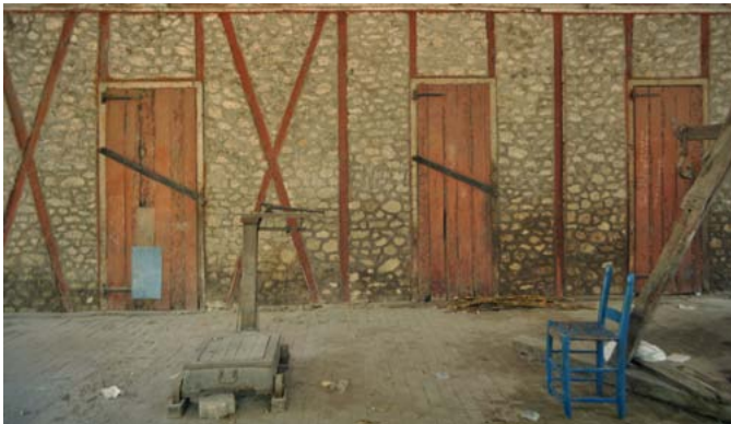
FIGURE 25 left A barn in Léogâne is an example of rubble stone colombage made with stronger igneous rocks than those used in Port-au-Prince, and not stuccoed. right A heavily damaged colombage wall showing the rubble stone infill characteristic of Port-au-Prince. See also figure 86.
