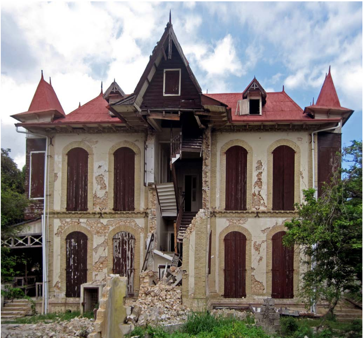
FIGURE 47 View of the back elevation of Castel Fleuri. The use of brick masonry surrounding the windows, at the corners, and at floor lines in tandem with the stucco over the stone masonry elsewhere forms a pleasing composition. Note the X-shaped end plates of the iron rods visible on the façade, which were not installed at the building corners in this case. See also Figure 108.
