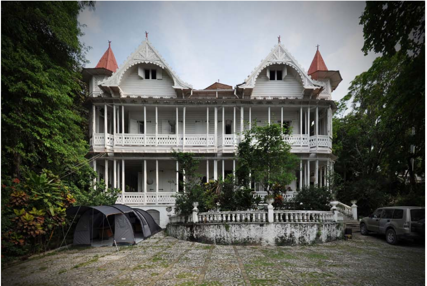
FIGURE 15 The 1912 Peabody House in Pacot. This colombage and timber frame house survived the earthquake almost undamaged.
