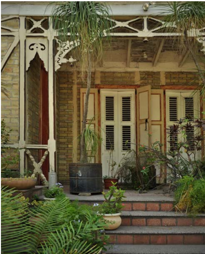
FIGURE 36 79 Avenue Christophe showing colombage with brick infilling.
