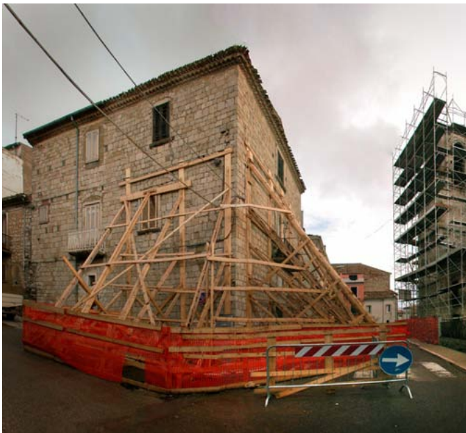
FIGURE 121 Examples of shoring in Italy after the Molise earthquake, showing the heavier timber diagonal braces in the example on the left, and polypropylene straps holding the building together on the right.
