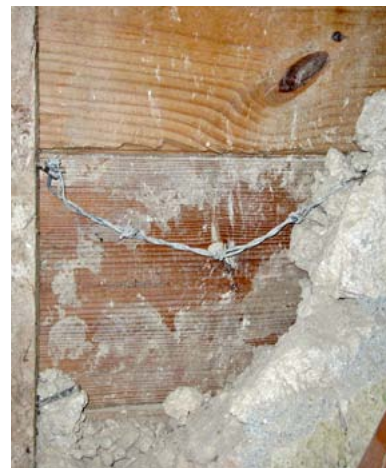
FIGURE 125 Barbed wire is frequently seen in the wall cavities as a restraint for the rubble fill. This is a good practice and should be continued.
