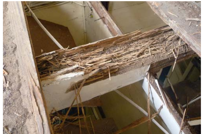
FIGURE 68 Termite damage in second story floor joists.
