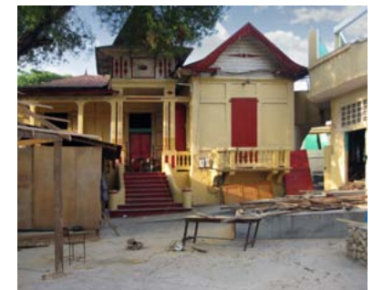
FIGURE 30 Concrete frame/confined masonry Gingerbread. This is the only variant of this type seen. It was undamaged.
