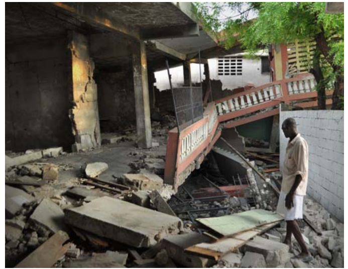
FIGURE 112 A small colombage school building at 16 Lamartiniere that had a two-story addition behind it. Large portions of this addition collapsed completely, but the original building is still intact and in use.
