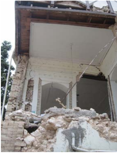
FIGURE 102 In this case the horizontal metal ties failed to prevent the collapse of these masonry walls, but may have helped prevent the collapse of the rest of the building
