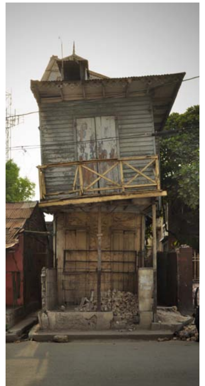
FIGURE 90 A wood clad and colombage structure of the most basic type on Rue Geffard near the National Palace. This structure appears to have been designed to be expanded to double its width, but never was. As a result, it was subject to the earthquake with a width at the base of less than 12 feet (3.6 meters). Also, at the time of the earthquake, it was in extremely poor repair. In spite of all of this, the earthquake did not cause it to collapse.
