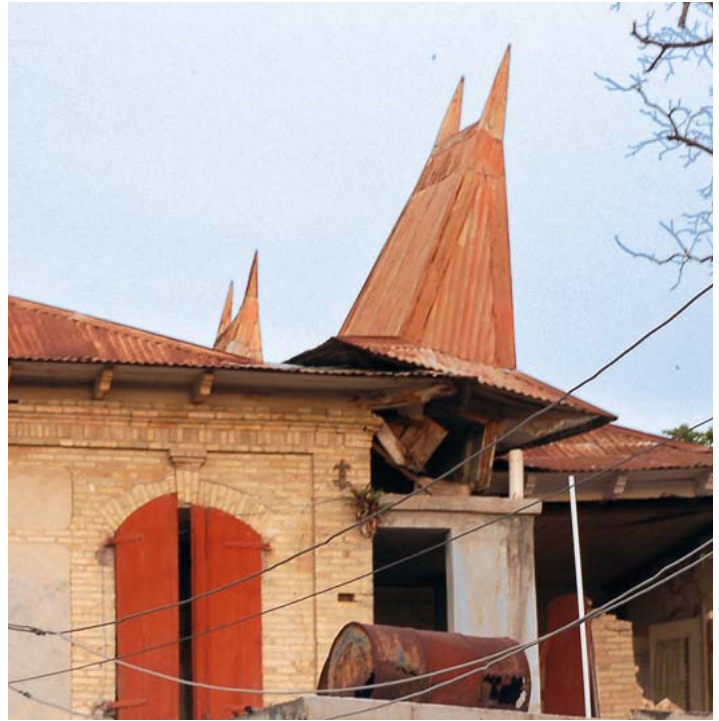
FIGURE 80 Both of the steeples of this Gingerbread house were shaken out of plumb during the earthquake.
