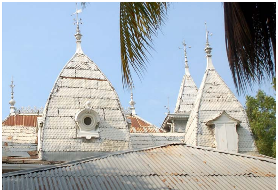
FIGURE 56 The roofs of the turrets of Le Manoir utilize decorative pressed metal roof shingles.
