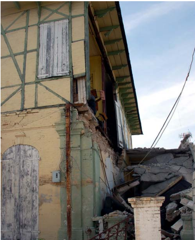
FIGURE 109 Interior and exterior of 51 Avenue Christophe showing reinforced concrete addition to the timber and colombage house. The two parts pulled away from each other during the earthquake.
