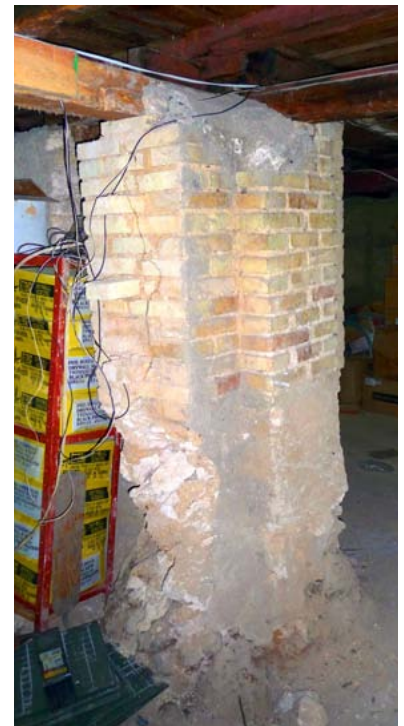
FIGURE 52 An excavated crawl space in the house at 84 Lamartiniere shows an original above-grade brick pier, and its uncovered, original limestone and earth mortar footing.
