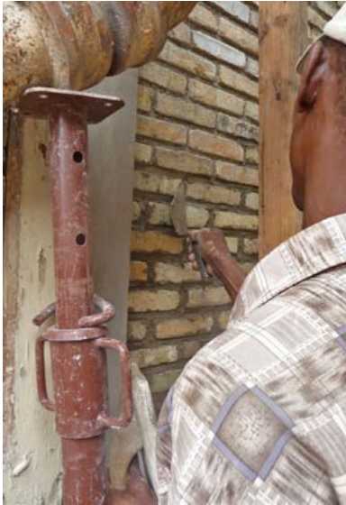
FIGURE 135 Well-intentioned but improper repairs with cement mortar in brick work ( above and right ), and cement plaster for colombage infill ( below ). Lime mortar and lime plaster should be used.
