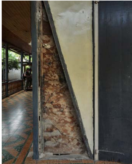
FIGURE 41 House at 15 Rue M showing plastered rubble stone infill. On the left, one panel fell out in the earthquake, revealing that it was reinforced with barbed wire inserted into the bay in a zigzag layout.
