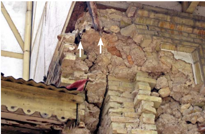
FIGURE 103 Embedded tie rods cross at the corner, anchored by iron bars. Also note rubble fill between inner and outer leaves of brick masonry.
