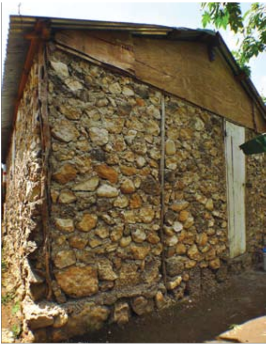
Timber frame house with stone-and-mortar infill.
