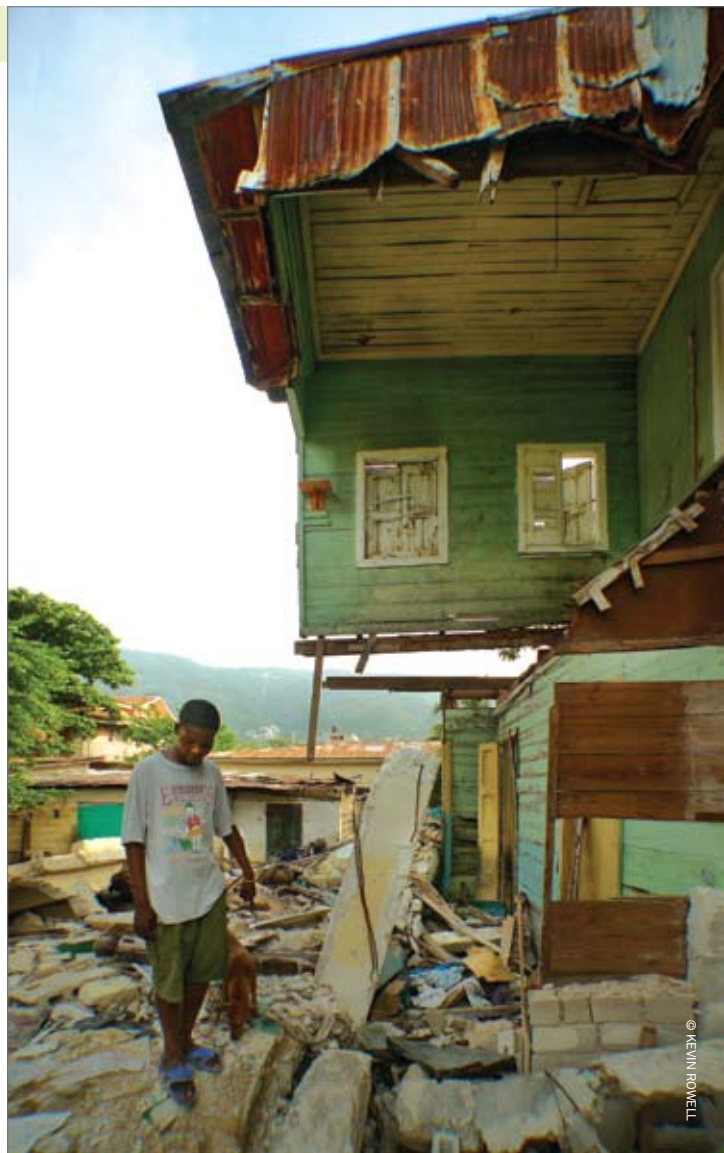
A concrete addition to this wood-frame house crushed and buried this man's cousin.
